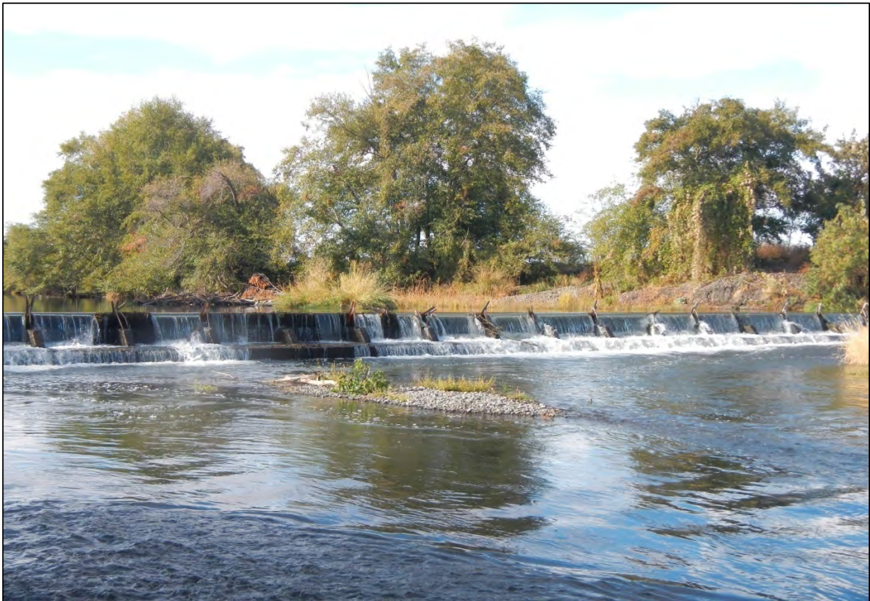
Figure 3-2. Site conditions during the October 24, 2012 site visit, 190 cfs. Photo is taken from the downstream river-right bank looking upstream at the structure. Note growth of gravel bar in foreground.
