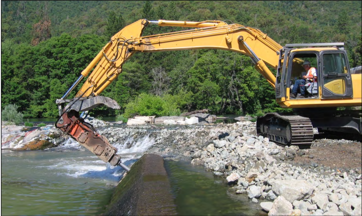
Figure 4-3. A trackhoe equipped with a pick for breaking concrete for removal.
