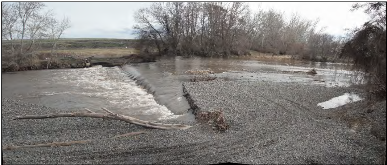
Figure 3-9. Photo of high flow conditions during March 2011 showing large amount of mobile sediment in the Umatilla River that deposits in and around the dam and illustrates the lack of influence the existing dam has on river processes.
