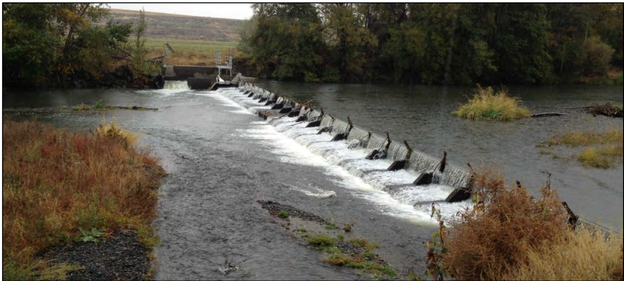
Figure 1-2. Existing Dillon Dam on the Umatilla River.
