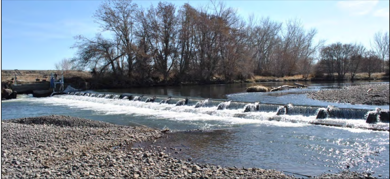
Figure 3-1. Site conditions during the March 7, 2012 site visit, 380 cfs. Photo is taken from downstream river-left gravel bar looking across the structure.
